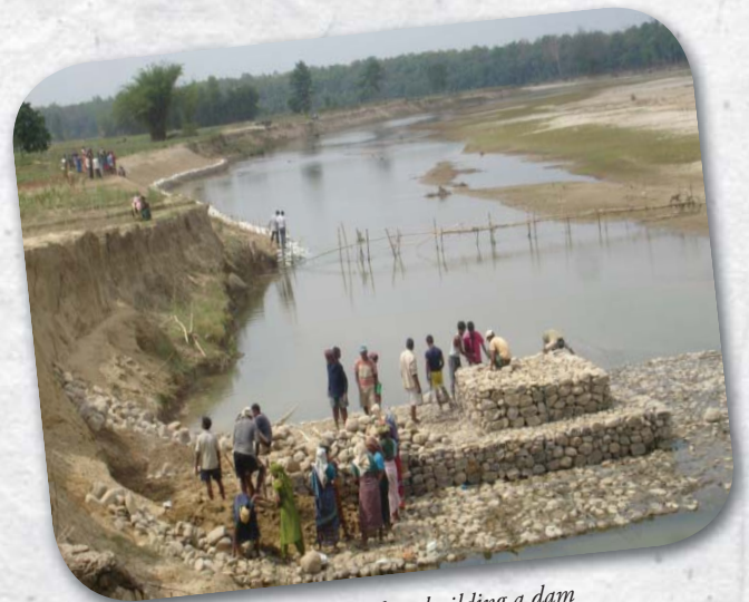
Community members building a dam
